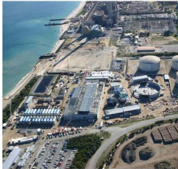
Figure 7-12: Perth SWRO Desalination Plant
