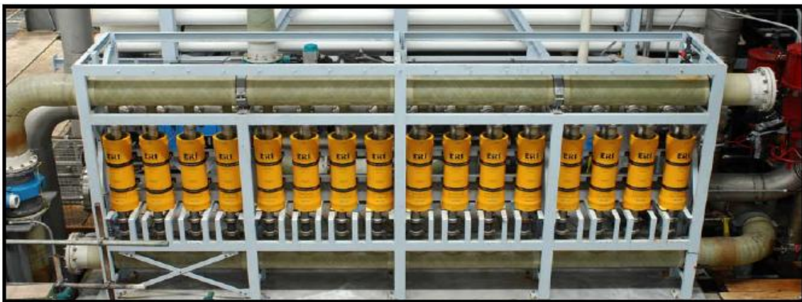
Figure 7-11: PX Device Array Serving SWRO Train 6A
